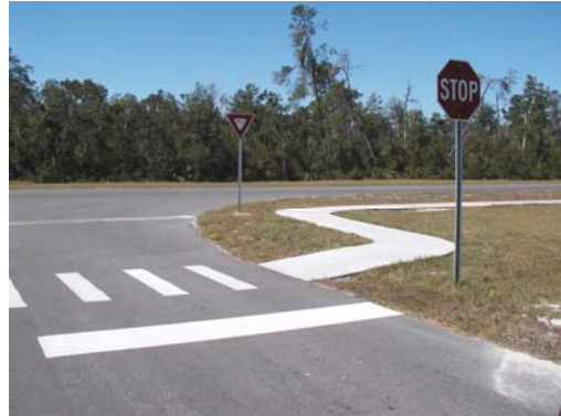
The crosswalk is located away from the intersection. Note the yield sign located at the intersection beyond the stop sign
