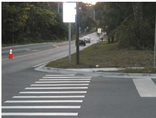
The new crosswalk at the school entrance road ends in a raised curb (missing ramp)
