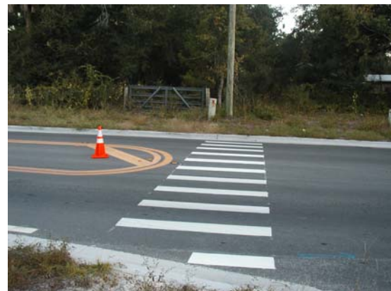
The crosswalk across Blue Springs Avenue leads to a constrained right of way with utilities. The curb ramp is also missing.
